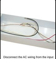
side of the ballast. Trim the AC wires
